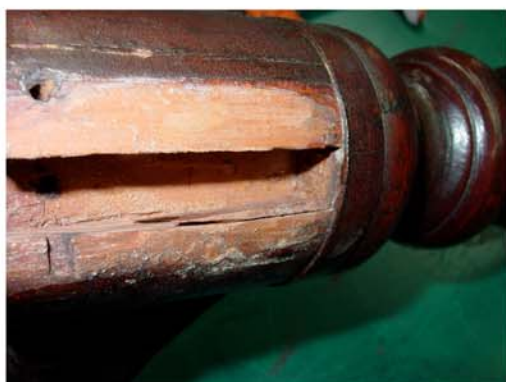
3A tripod repair (37)
