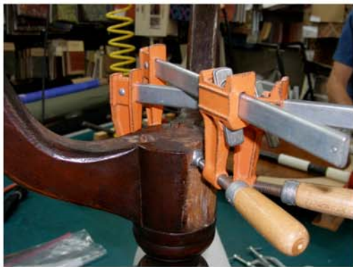
3A tripod repair (14)
